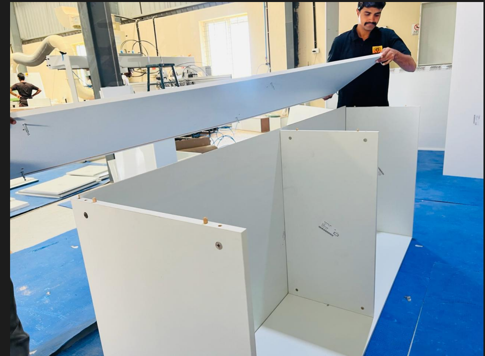
PRE-INSTALLATION AT FACTORY
